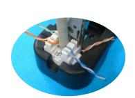
Punch the wires with 110 or Krone impact tool and cut off the surplus wires.
